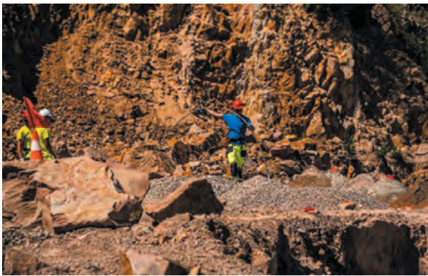
Fig. 8. Blasting works performed by SSE
