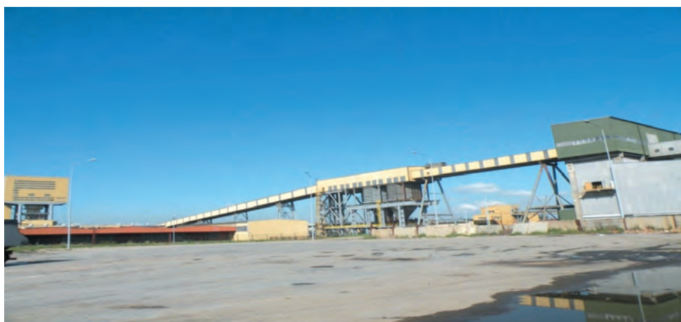
Fig. 19. Rock salt and copper ore conveyor belt
