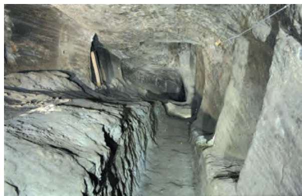
Fig. 3. Traces of salt blocks loosening (phot. by Adam Brzoza)
