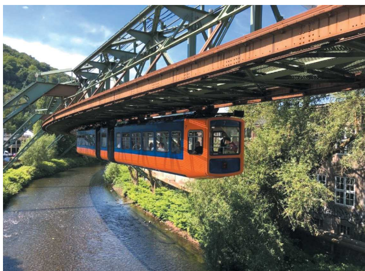
Fig. 4. Wuppertaler Schwebebahn railway [3]
