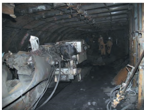
Fig. 20. Longwall closure drift secured by means of the ŁPro/B support
