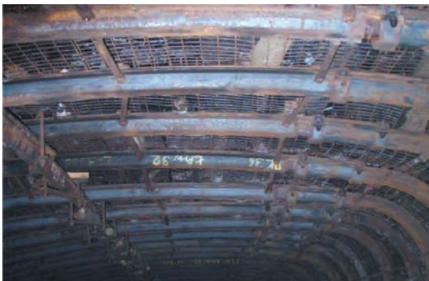
Fig. 47. Development drift secured by means of the ŁPrw support
