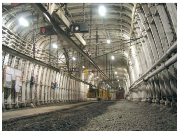
Fig. 44. Railway station constructed inside an ŁPrP variant Ł support
