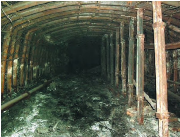
Fig. 33. Development drift secured with four-element ŁPrP frames
