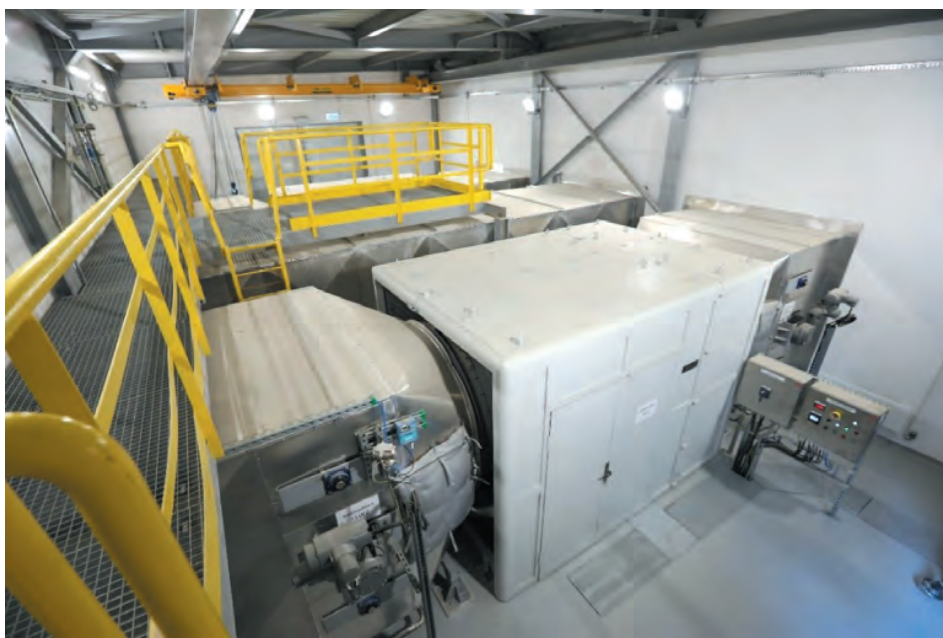
Fig. 5. “Wilson” shaft after retrofitting (phot. R. Stachurski)
