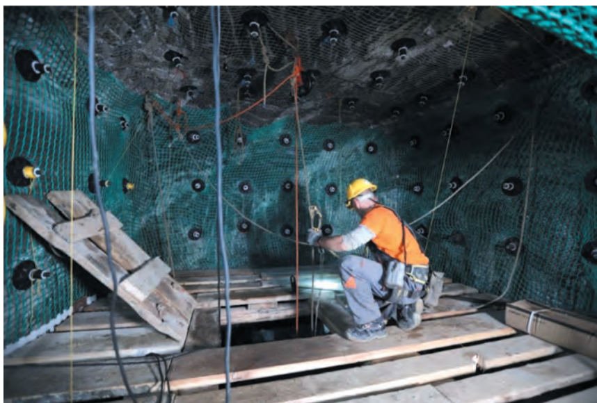
Fig. 6. Works carried out in “Geramb” shaft (phot. R. Stachurski)
