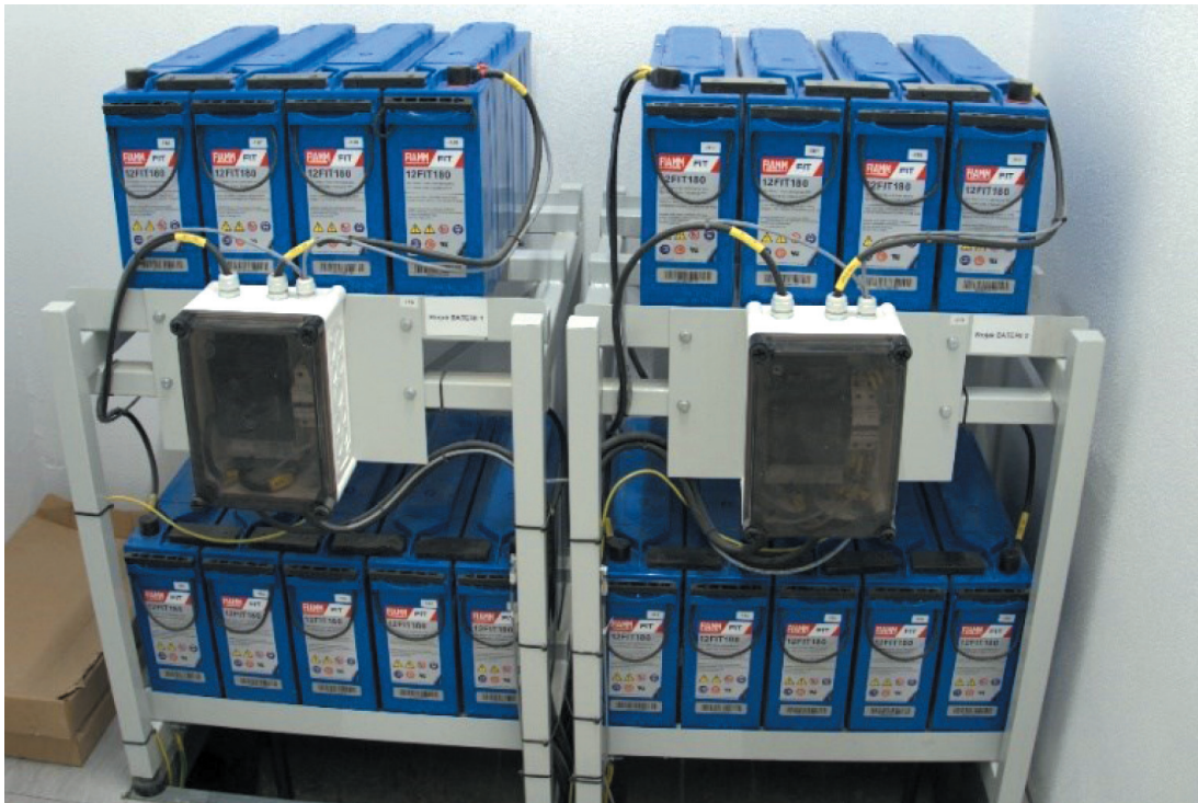
Fig. 8. Accumulator batteries
