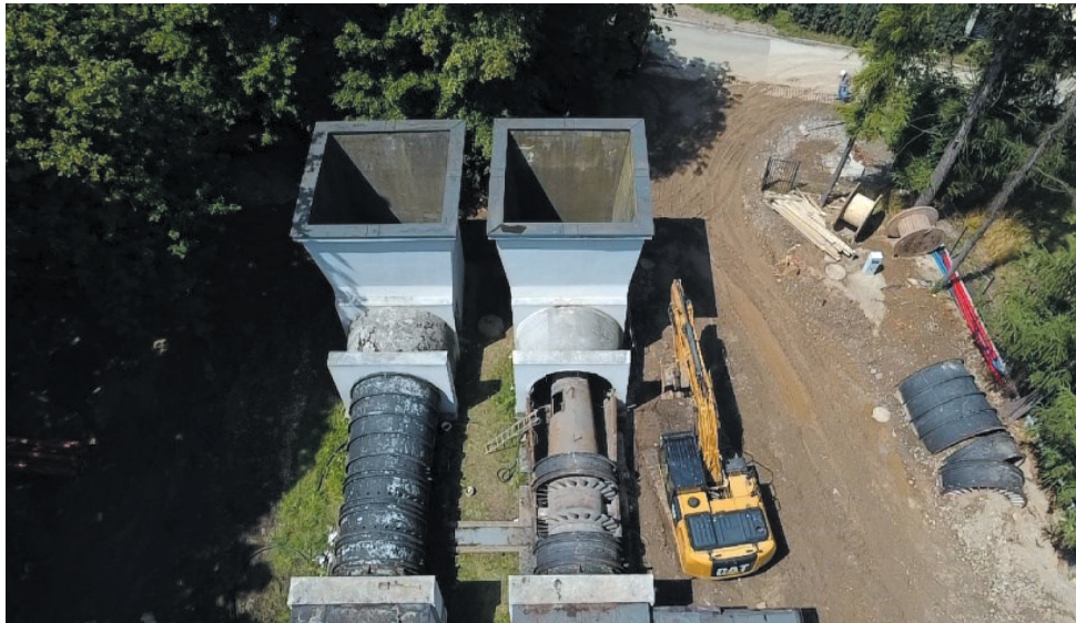
Fig. 1. Main ventilation fans for “Wilson” shaft
